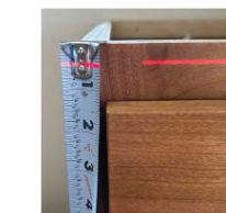
At measure - laser shows unlevel cabinets greater than 1/4"
