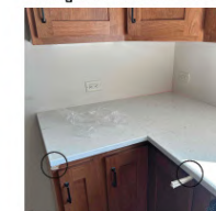
Countertop sitting on shims to level with highest cabinet
