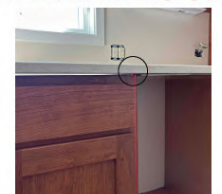
Cabinet lower than starting point 1 shim needed
