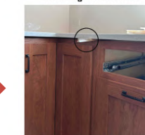
Continuation of cabinets unlevel 3 shims used
