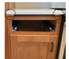
Lowest cabinet and most unlevel from the highest cabinet - several shims needed
