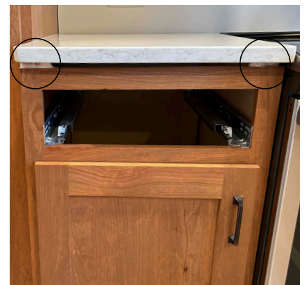
Lowest cabinet and most unlevel from the highest cabinet - several shims needed
