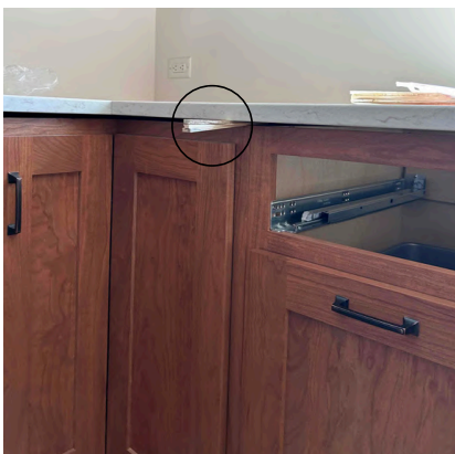
Continuation of cabinets unlevel 3 shims used
