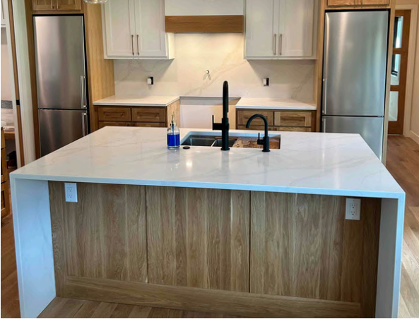
EXAMPLES OF WATERFALL EDGE CUT FROM THE SAME SLAB
