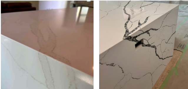
EXAMPLES OF WATERFALL EDGE CUT FROM THE SAME SLAB
