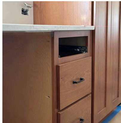
Countertop set on highest cabinet, sitting flush on cabinet - no shims
