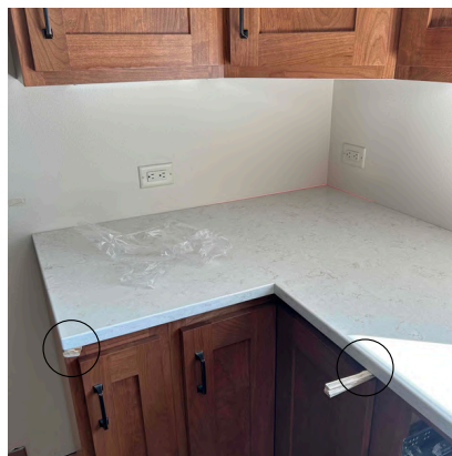
Countertop sitting on shims to level with highest cabinet
