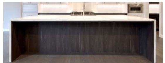
EXAMPLES OF CABINET PANELS USED TO COVER THE BACKSIDE OF THE WATERFALL UNFINISHED BACKSIDE
