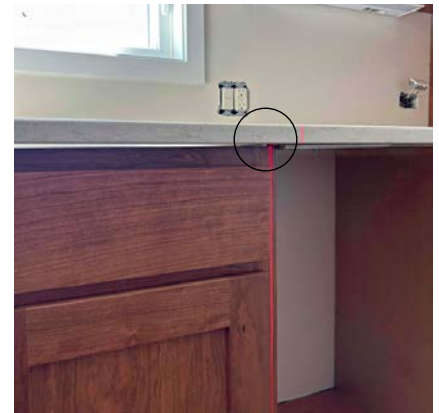
Cabinet lower than starting point 1 shim needed
