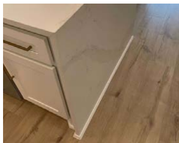
EXAMPLE OF WATERFALL EDGE INSTALLED TO SUBFLOOR/NOT LVP NOTICE 1/4 ROUND TO COVER GAPS
